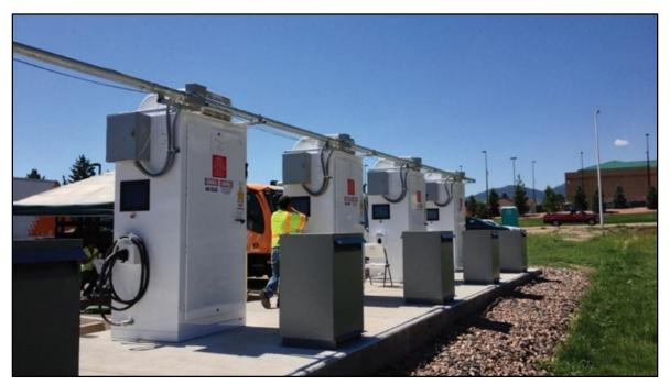
This is an example of distributed microgrid controllers. In this case, the controllers are the grey boxes installed beside these bidirectional electric vehicle chargers on a military base in Colorado.
